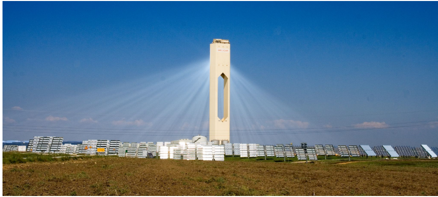
Figure 1.1: PS10 solar power plant, central receiver system located in Andalusia, Spain. The heliostat field focuses sunlight onto a tower-mounted receiver, where heat is collected for storage and electricity generation. 1
